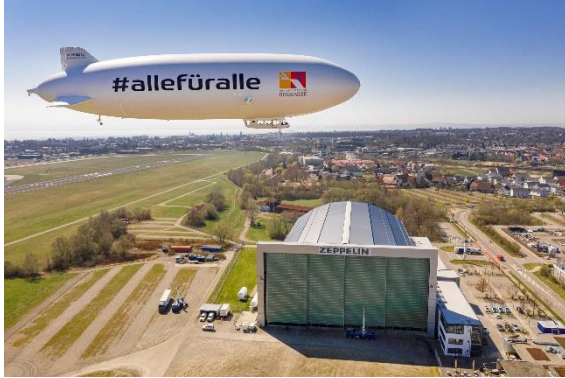
Zeppelin hangar © Michael-Haefner
