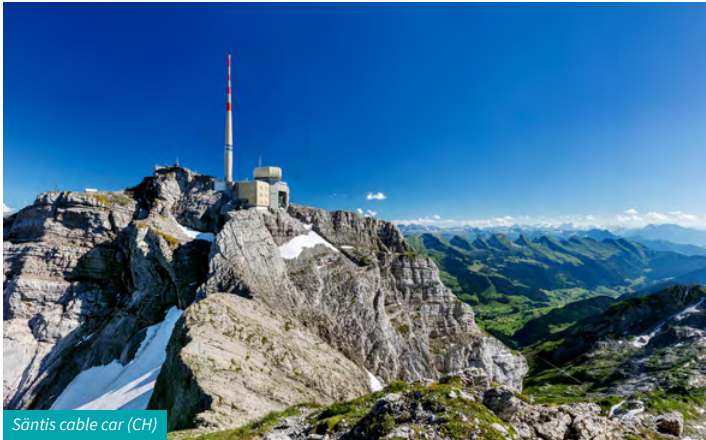
Säntis cable car (CH)
